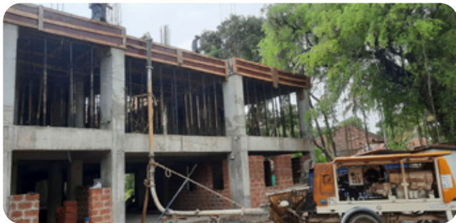
Columns on the ground floor raised.
