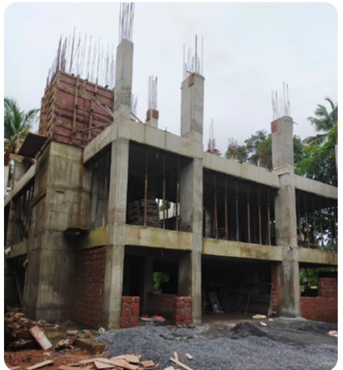
Concreting of columns of the first floor slab completed.
