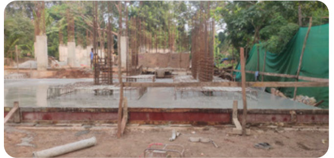
All hands on deck and 80% of the foundation laid.
